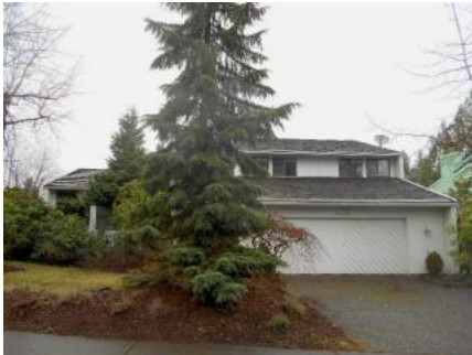
17521 155th Ave Se, Renton, WA 98058
