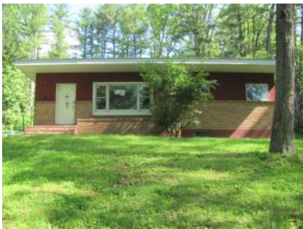
1424 River Rd, Binghamton, NY 13901
