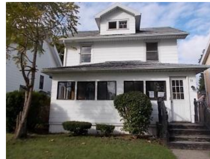
72 Culver Parkway, Irondequoit, NY 14609
