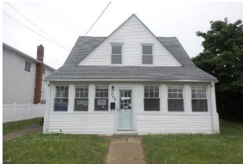
208 Rhame Avenue, East Rockaway, NY 11518
