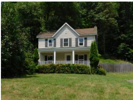
112 Route 55, Warwarsing, NY 12458
