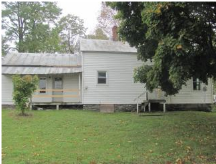
917 County Highway 49, Pittsfield, NY 13411
