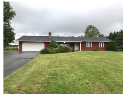
10678 Mile Block Road, North Collins, NY 14111
