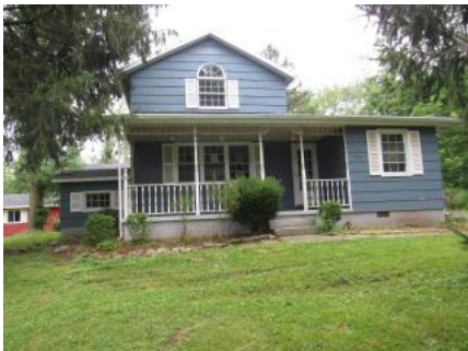
306 Plank Road, Lockport, NY 14094
