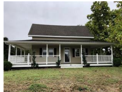
62 Newport Rd, Newport, NJ 08345
