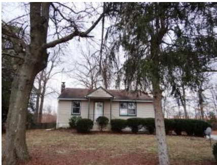
750 Hawks Bridge Rd, Salem, NJ 08079
