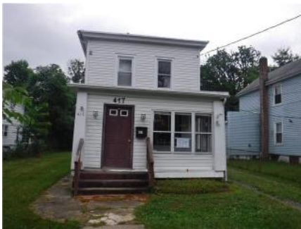
417 S East Avenue, Vineland, NJ 08360
