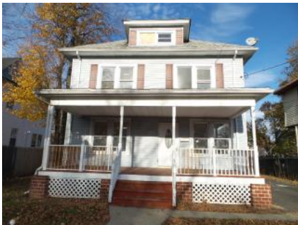
135 Johnston Ave, Plainfield, NJ 07062
