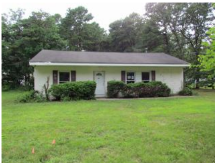
445 Prince Avenue, Williamstown, NJ 08094
