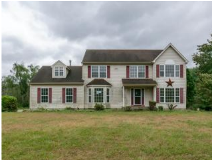
100 Spring Hill Dr, Woolwich Township, NJ 08085
