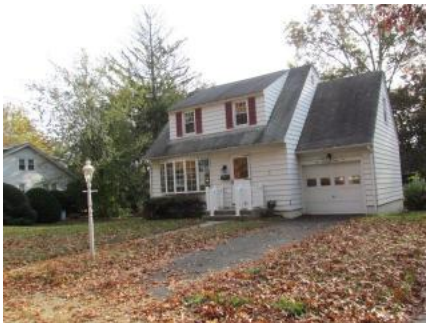
561 High Street, Woodbury, NJ 08096
