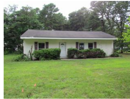
445 Prince Avenue, Williamstown, NJ 08094
