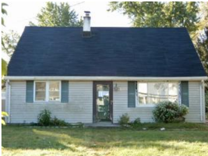
209 Eaton Ave, Hamilton, NJ 08619
