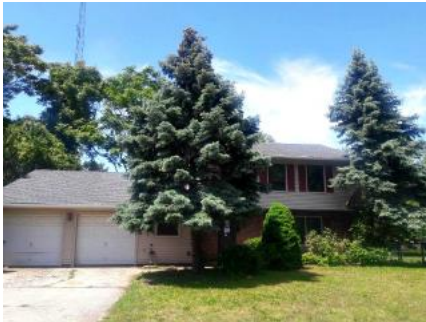
18 Ash Rd, Edison, NJ 08817
