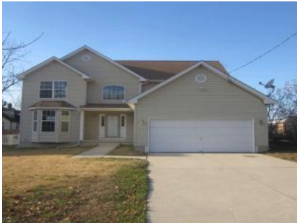
101 Pennsylvania Ave, Clementon, NJ 08021
