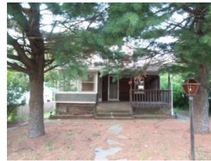
37 East Gloucester Pike, Barrington, NJ 08007
