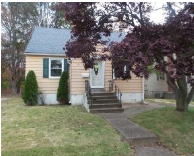
439 E Park Avenue, Maple Shade, NJ 08052
