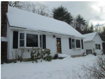
540 Catamount Rd, Pittsfield, NH 03263
