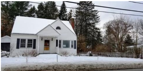
25 Portland St, Lancaster, NH 03584
