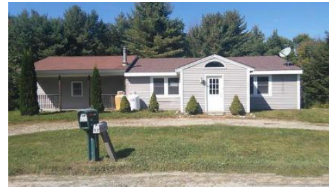
82 Quaker City Road, Unity, NH 03773
