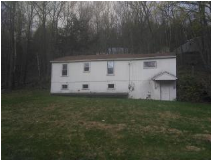
26 Pumping Station, Lebanon, NH 03766
