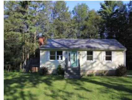
6 Laurel Lane, Stafford Springs, CT 06076
