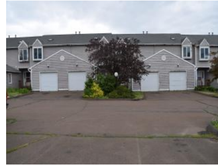
255 Pine Rock Ave Unit 13, Hamden, CT 06514
