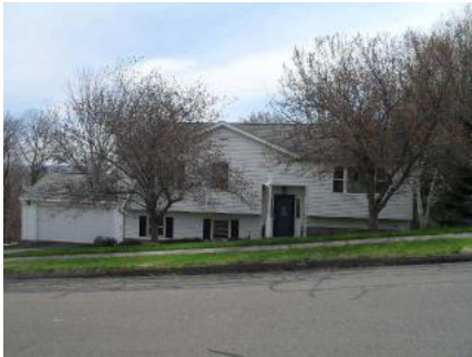
59 Cimarron Road, Middletown, CT 06457
