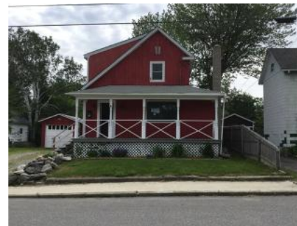
84 Bannon Street, Torrington, CT 06790
