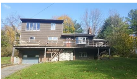
109 Lower Road, East Canaan, CT 06024
