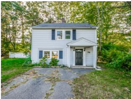
74 Colorado Ave N, Torrington, CT 06790
