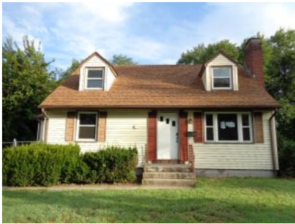
131 Collins Road, Bristol, CT 06010
