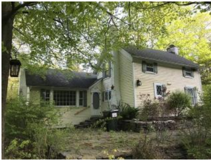
357 State Route 37, New Fairfield, CT 06812
