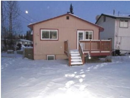
116 North Lane Street, Anchorage, AK 99508
